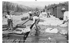
each end of the cars. Rock salt was sprinkled in to lower the melting point of the ice, kind of like making iced cream in a hand crank iced cream maker. The roof hatches on the roof had a prop rod with notches that allowed the hatches to be kept open and allow some
