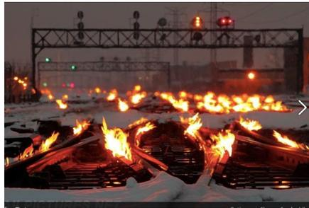
today's heaters are that they can operate over a long time, and many can be started and shut off remotely. Track insulation can be applied to the rails to minimize the heat loss. Rails only need to be warmed to just above freezing to be effective.
